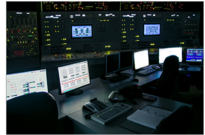
PEPSE provides integrated performance data and the means to construct detailed system models
