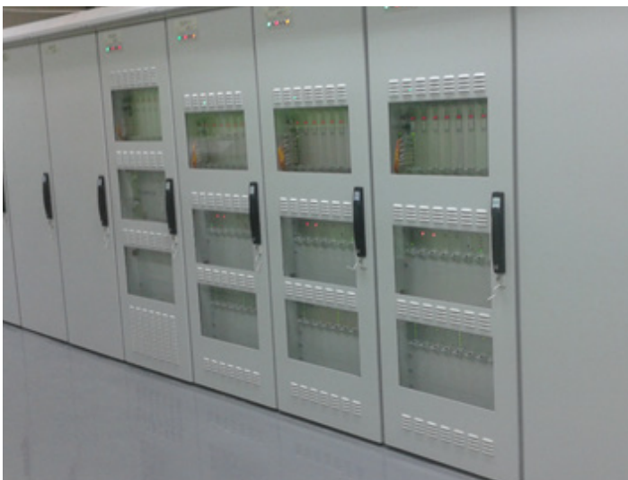
South Ukraine NPP (Unit 3) Reactor Trip System
