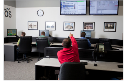
Image of Monitoring and Diagnostics Center
